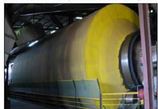
Figure 3 Three-pass rotary drum drying process in the ITPS DÉSRY dehydration site of Toulouse.
